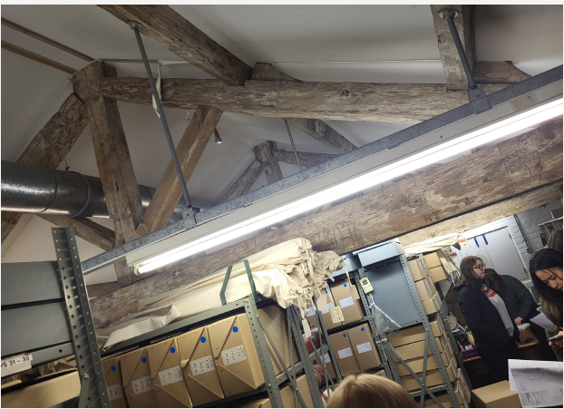
High ceilings and Exposed beams
